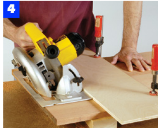
After gluing up the panels, use a circular saw to cut the panels to size with the appropriate angled ends and edges.
